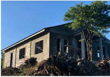
Church Construction Progress in Labney
